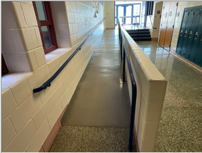
ACCESSIBLE INTERIOR RAMP
