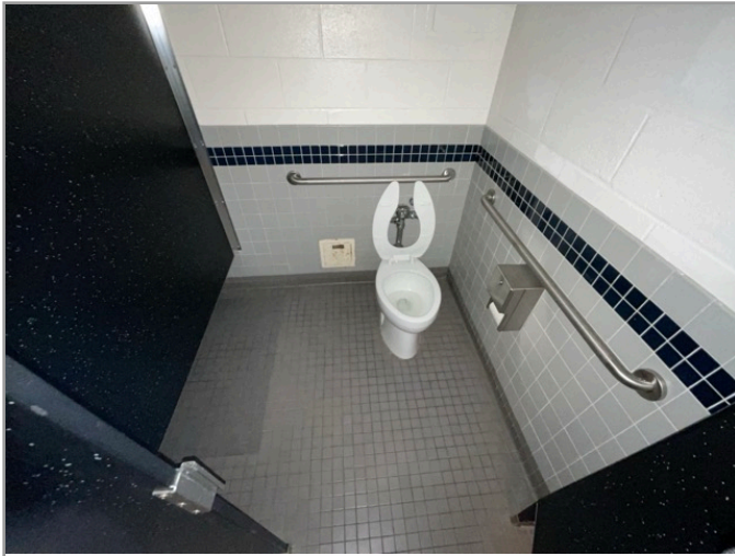
TOILET STALL OVERVIEW
