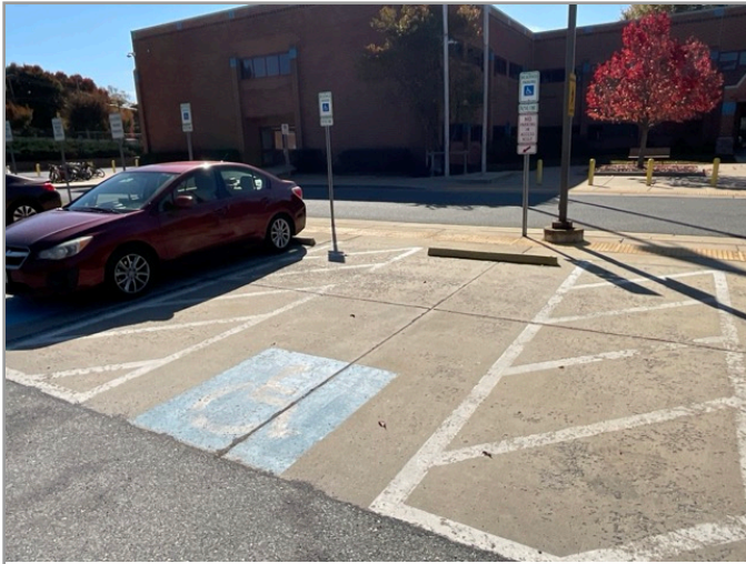
OVERVIEW OF ACCESSIBLE PARKING AREA
